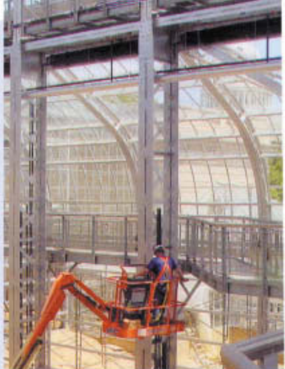
Rough Brothers completely restored the USBG's Palm House.
