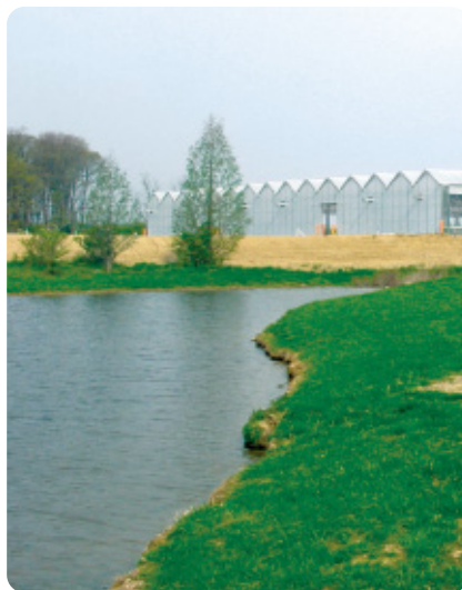
With the increasing concern for environmental issues and the enforcement of protective regulations, more growers are adding a holding pond.
